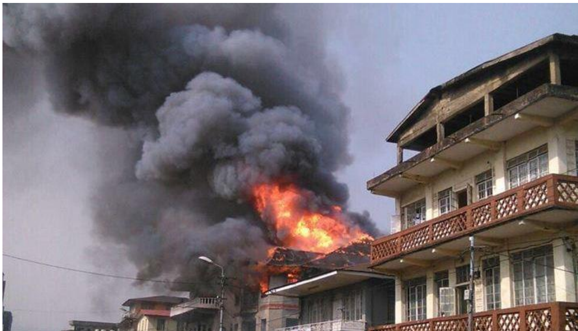
Figure 5-13: Fire disaster events in Freetown, Sierra Leone – 19 February 2016
